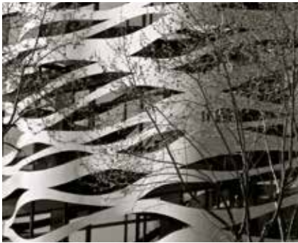
Facade renovation of Suites Avenue Aparthotel by Toyo Ito, Barcelona, Spain, is biomorphic in form, while enhancing the Dynamic & Diffuse light and shadows filtering to the interior space. Image © Aslaj/Flickr.
